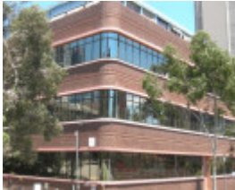
RMIT BUILDING NO. 9 SOHE 2008
