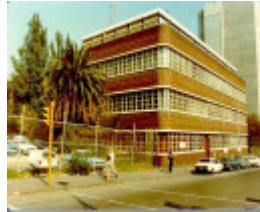
1 rmit building no 9 rear view 1982
