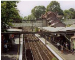
B7220 Camberwell Railway Station
