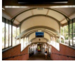
B7220 Camberwell Railway Station
