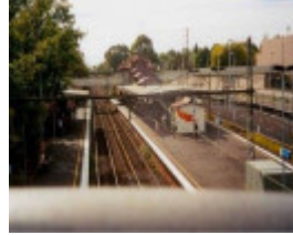
B7220 Camberwell Railway Station
