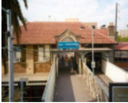
B7220 Camberwell Railway Station
