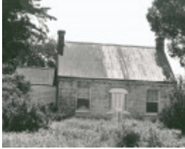
B3360 Cottage Forrest Rd South Corio
