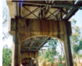
B7277 Bridge over Sunday Creek
