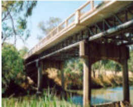
B7277 Bridge over Sunday Creek
