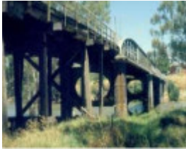
B7296 John Foord Bridge
