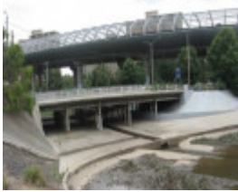
B7312 Flemington Bridge
