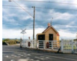
B7315 New St Railway Gates
