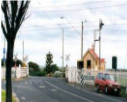
B7315 New St Railway Gates
