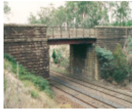
B7318 Middle Gully Bridge
