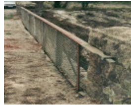
B7318 Middle Gully Bridge
