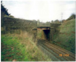
B7319 Harper's Lane Bridge
