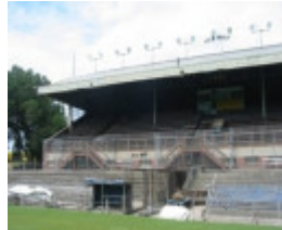
B7350 North Melbourne Grandstand
