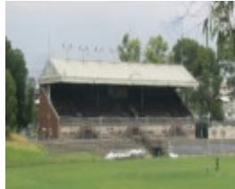
B7350 North Melbourne Grandstand
