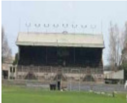
B7350 North Melbourne Grandstand
