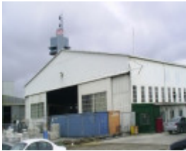
B7360 Fmr Comm Aircraft Hangar Site
