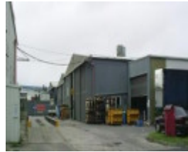
B7360 Fmr Comm Aircraft Hangar Site
