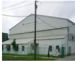
B7360 Fmr Comm Aircraft Hangar Site
