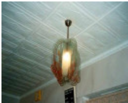
B7344 Lobby Ceiling
