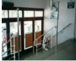
B7344 Entry Stairs
