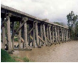
B7371 Latrobe River Bridge
