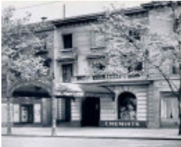
ogg & company demolished 76 collins street front view
