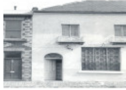
B1629 Queens Arms Hotel South Melbourne
