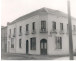
B1629 Queens Arms Hotel South Melbourne
