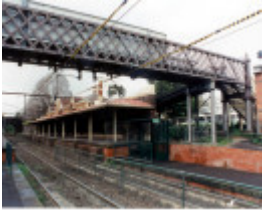
B4794 South Melbourne Station
