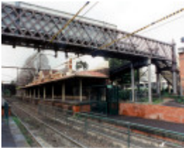
B4794 South Melbourne Station
