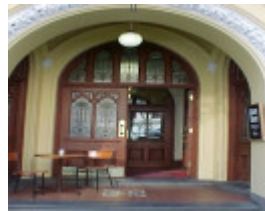
professional chambers collins street melbourne entrance detail sep1999
