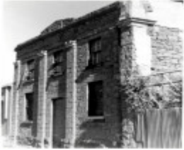
B1671 Methodist Sunday School Building Brunswick St Fitzroy
