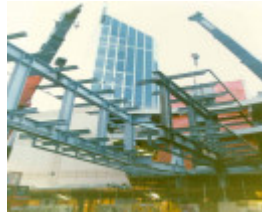
B5065 Lonsdale St Footbridge
