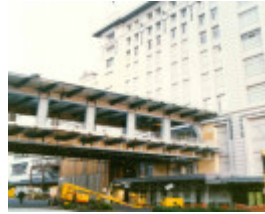
B5065 Lonsdale St Footbridge
