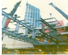
B5065 Lonsdale St Footbridge
