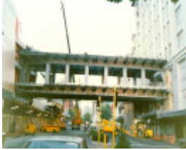
B5065 Lonsdale St Footbridge
