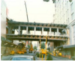
B5065 Lonsdale St Footbridge
