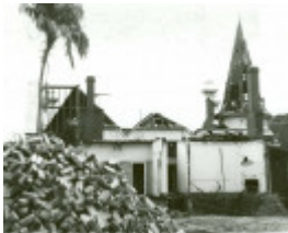
B4787 Koonwarra Demolition
