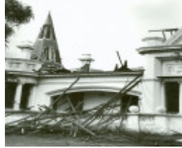
B4787 Koonwarra Demolition
