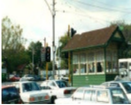
B6853 Tram Shelters St Kilda Rd & High St & Lorne
