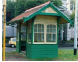
B6853 Tram Shelters St Kilda Rd & Dorcas St
