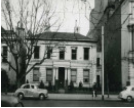
B0080 19 Collins Street .jpg
