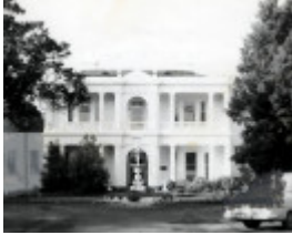
B1533 Armadale 461 St Kilda Rd Melbourne
