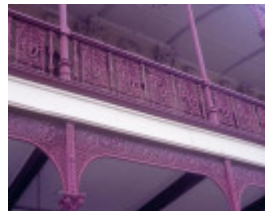
h00116 old colonists hall lydiard street north ballarat iron lace work she project 2004
