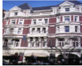
1 austral building collins street melbourne front view
