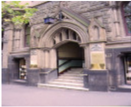
assembly hall collins street melbourne entrance detail feb1993
