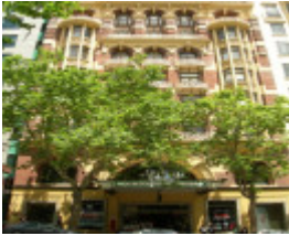
FORMERLY THE AUDITORIUM SOHE 2008
