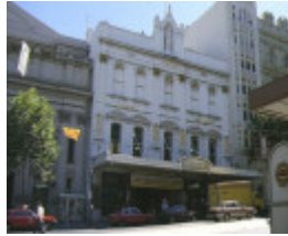
1 the athenaeum building collins street melbourne street view feb1986
