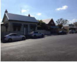
Falls Road Precinct
