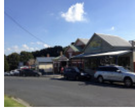
Falls Road Precinct
