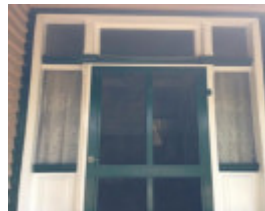
Front entrance door, 14 Bridge St
