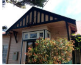
'Flying' gable, 14 Bridge St
