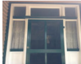
Front entrance door, 14 Bridge St
