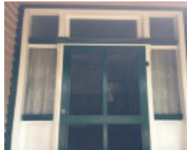
Front entrance door, 14 Bridge St
