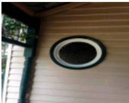
Porthole window, 14 Bridge St
