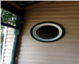
Porthole window, 14 Bridge St
