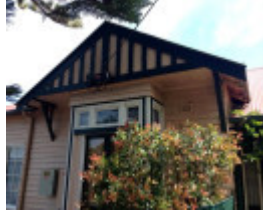
'Flying' gable, 14 Bridge St
