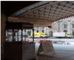
regent theatre collins street verandah detail jul1999
