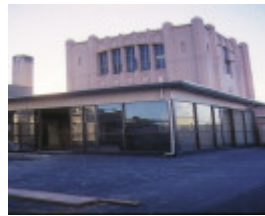
manchester unity building collins street melb roof building
