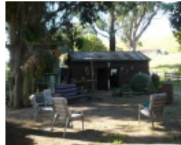
Outbuilding in rear yard of house, 1790 Grand Ridge Rd
