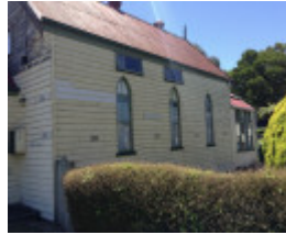
Bena Presbyterian Church (south elevation)
