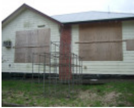
Bena School (former)
