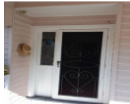
House, 21 Bridge Street
