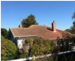
House, 21 Bridge Street
