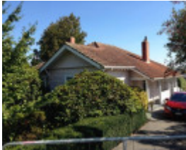
House, 21 Bridge Street
