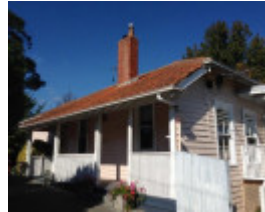
House, 21 Bridge Street
