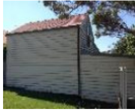
St Austell, stables
