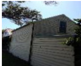
St Austell stables
