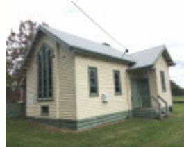
St Mark's Church of England (former)
