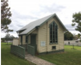
St Mark's Church of England (former)
