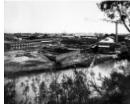
1918 - Yarra Falls construction.jpg
