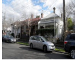
Late Victorian and Federation houses at 32-36 Charles St (recommended for inclusion in HO319)
