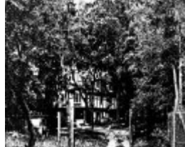
Ross House - 50 Arthur Street, Eltham
