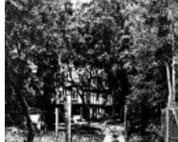
Ross House - 50 Arthur Street, Eltham
