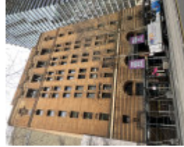
Former AMP Building - northern elevation - July 2021
