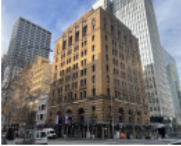
Former AMP Building July 2021
