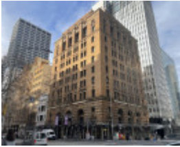
Former AMP Building July 2021
