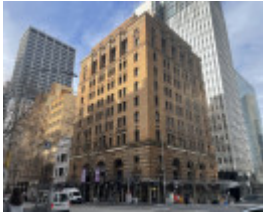
Former AMP Building July 2021
