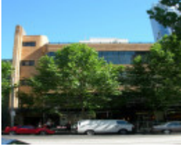
FORMER MCPHERSONS BUILDING SOHE 2008
