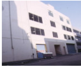
former mcphersons building collins street melbourne rear view
