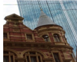
winfield building collins street melbourne turret detail sep1999
