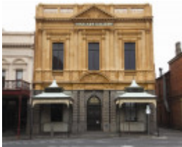
BALLARAT ART GALLERY_Restored Facade_Compressed.jpg 2010
