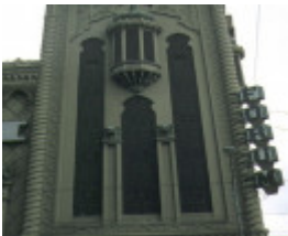
former state theatre flinders street melbourne external detail side sign
