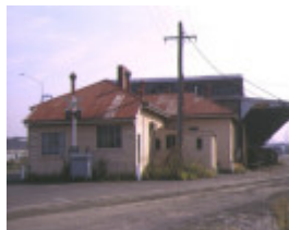
exhibition goods shed spencer street melbourne amenity room number 6 shed mar1989
