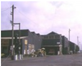
exhibition goods shed spencer street melbourne remnants of number 1 shed
