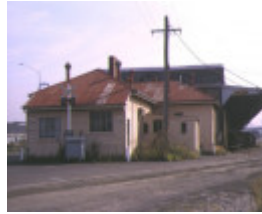
exhibition goods shed spencer street melbourne amenity room number 6 shed mar1989
