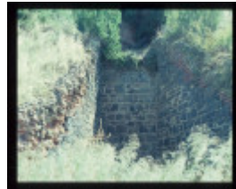
OLD STEIGLITZ ROAD BRIDGE
