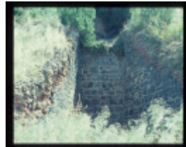
OLD STEIGLITZ ROAD BRIDGE
