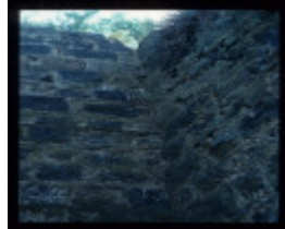
OLD STEIGLITZ ROAD BRIDGE FEATURE
