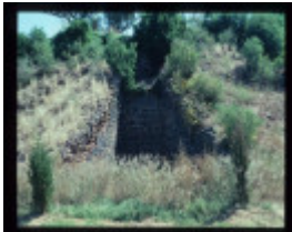
OLD STEIGLITZ ROAD BRIDGE
