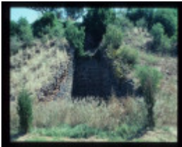
OLD STEIGLITZ ROAD BRIDGE
