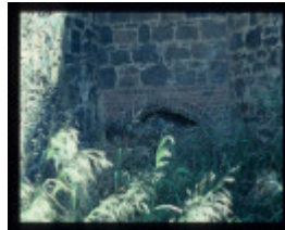
OLD STEIGLITZ ROAD BRIDGE FEATURE
