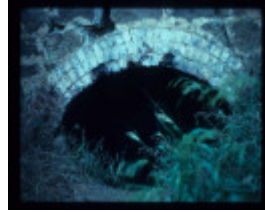
OLD STEIGLITZ ROAD BRIDGE FEATURE
