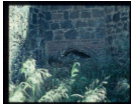
OLD STEIGLITZ ROAD BRIDGE FEATURE
