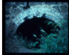
OLD STEIGLITZ ROAD BRIDGE FEATURE
