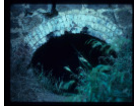
OLD STEIGLITZ ROAD BRIDGE FEATURE
