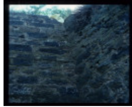
OLD STEIGLITZ ROAD BRIDGE FEATURE
