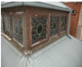
Before Photograph - Reference F3907 2014
