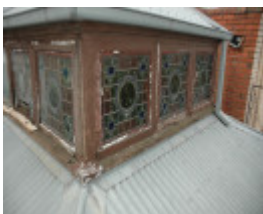
Before Photograph - Reference F3907 2014
