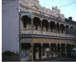
1 reids coffee palace ballarat front view yellow facade
