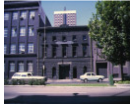
1 former zanders no3 warehouse king street melb street view
